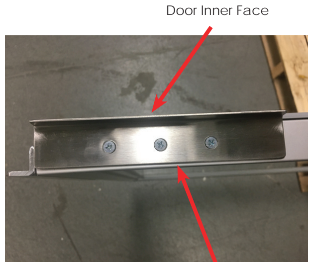
Fig. 49: Proper position of Cam Lock
