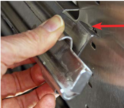
Fig. 20: Inserting Top Channel Tab
