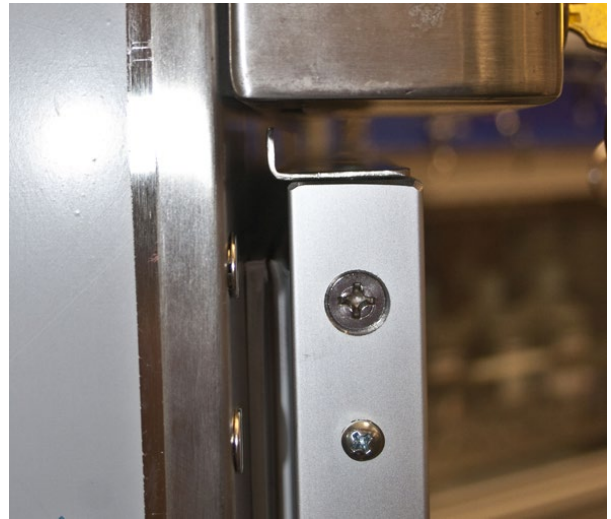
Fig. 51: Cam Lock Plate door gap
