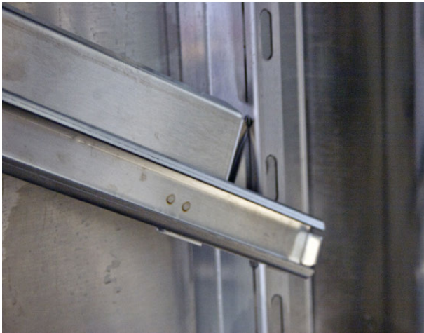
Fig. 14: Set Rail in New Position
